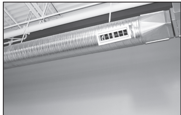
Drum louver shown in an open ceiling gym environment
