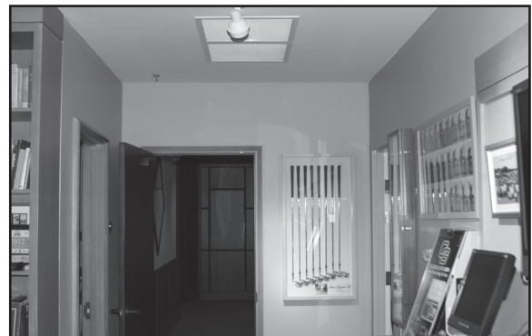
Installation image of the 45F Eggcrate Return Grille installed in a gift shop
