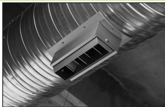
Installation images of the S-DL drum louver installed in an open ceiling environment
